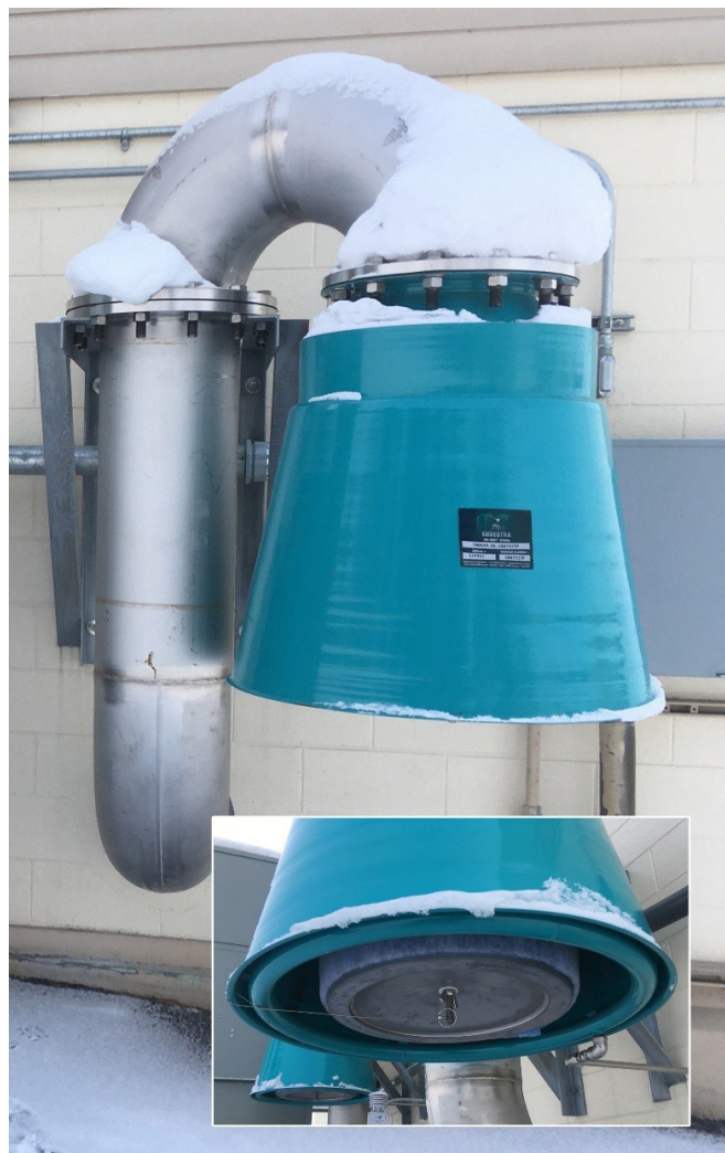
The Tri-Vent® Series TM09 with freeze discouragement discharge-air knife was designed to use waste heat generated by air compression.
