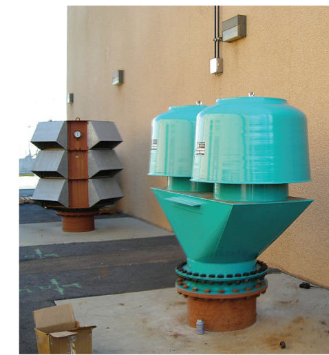
↑ Intake filter silencer installed next to an older style pane filter
